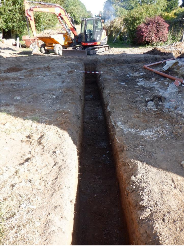
Plate 6. Foundation trenches (looking NW)
