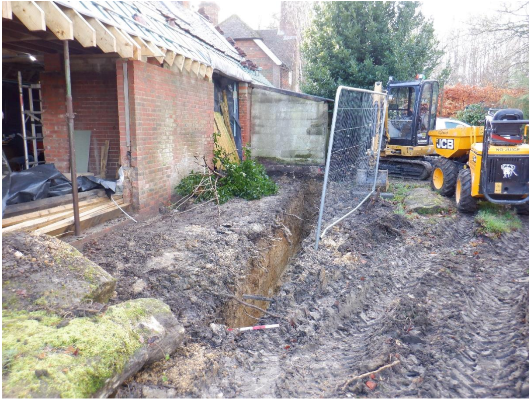
Plate 2. View of foundation trenches (looking NNW)
