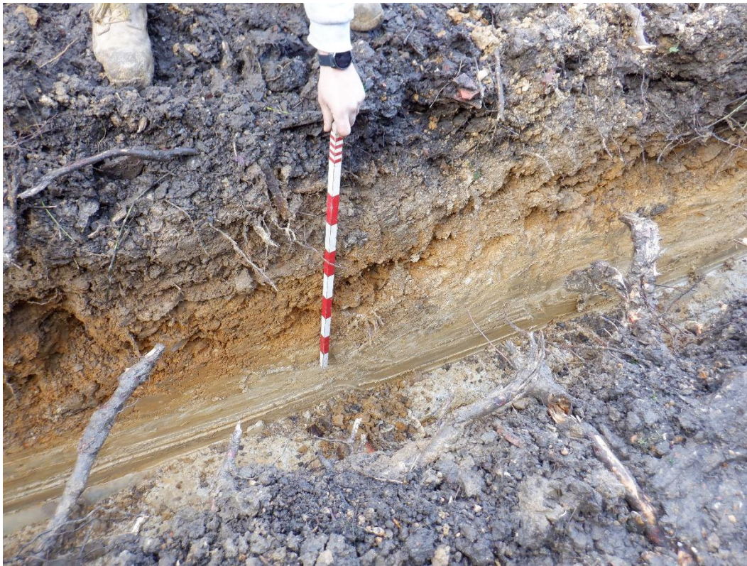
Plate 3. View of foundation trenching (looking W)
